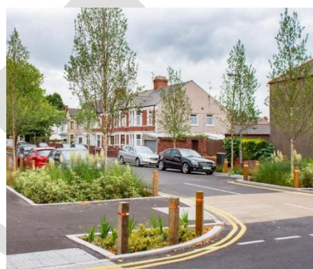
Kerbside raingardens, Cardiff
